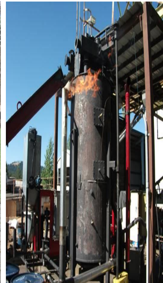
Fluidyne Pacific Class Gasifier
