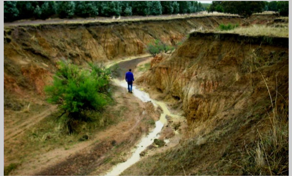
Approximately 280,000 tonnes of soil have eroded from this one kilometre section of the Crawford River in south-west Victoria since 1850, at a rate of approximately 5 tonnes per day. There are many rivers in similar condition throughout Australia.
